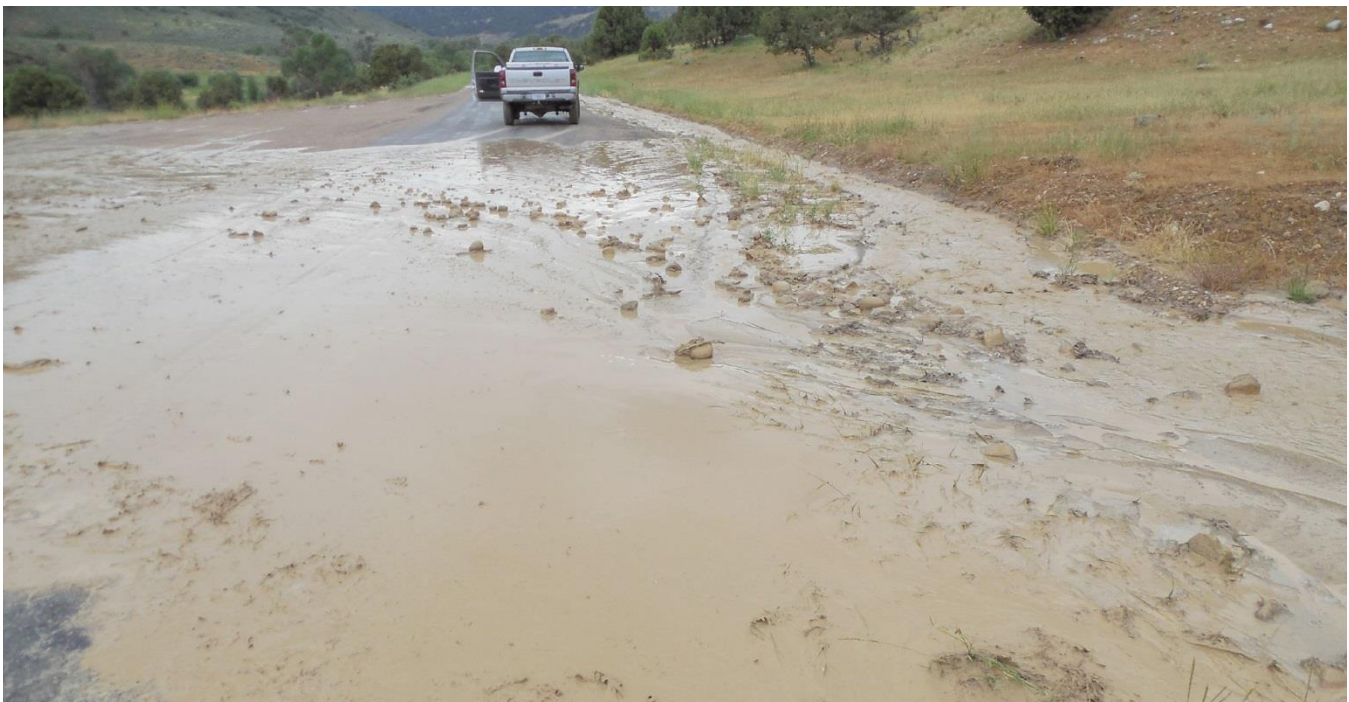
Just after a rainstorm, sediment from the hillsides covering the county road, the primary access to the watershed.
